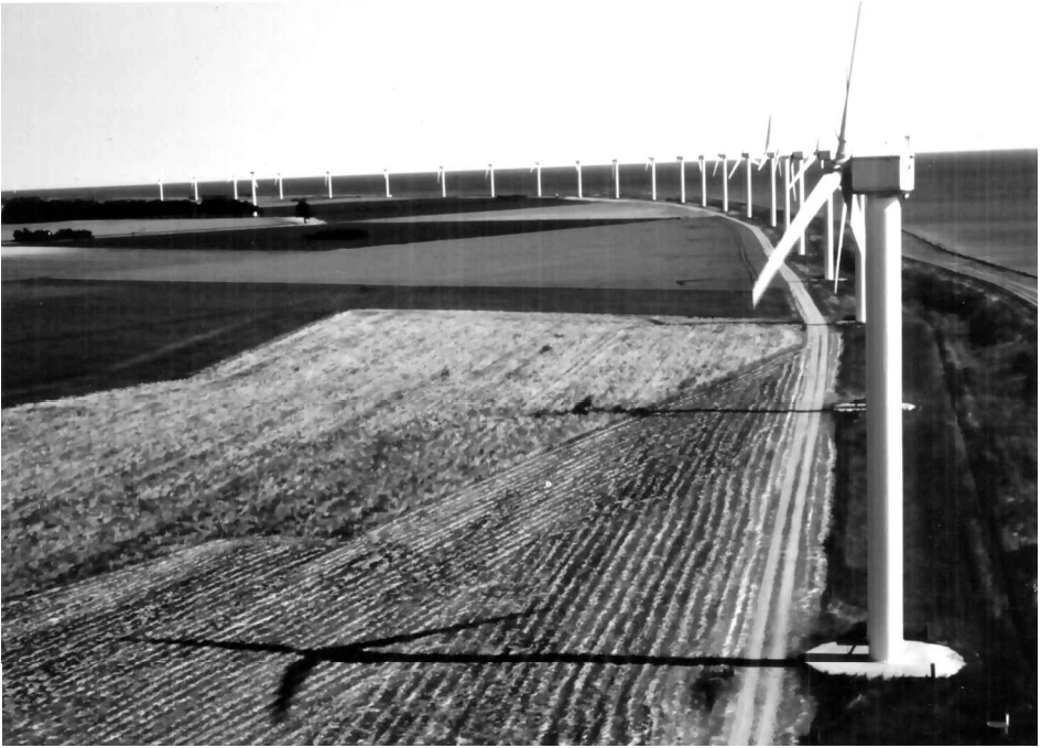
FIGURE 4 Deployment of wind turbines along the coast at Kappel, Denmark, displaying conformity and uniformity. The 24 turbines, commissioned in August 1990, have a capacity of 9.6 MW. Photo by Jens Bygholm, used with permission.
