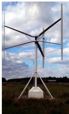
Figure 1. The 12 kW turbine, designed and built by the Division of Electricity at Uppsala University. The turbine is equipped with load cells used for the force measurements [31]
