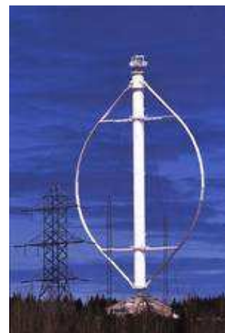
Fig. 13. Éole, the world largest Darrieus wind turbine.
