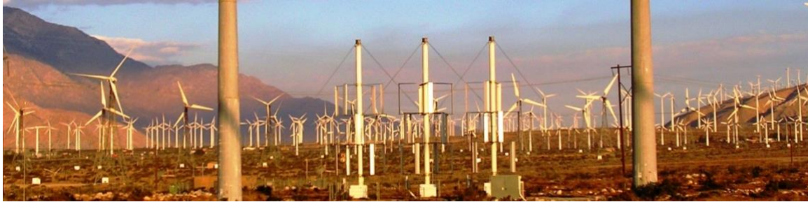
Three Windstar 530G VAWTs among HAWTs in the San Geronio Wind Resource Area , California
